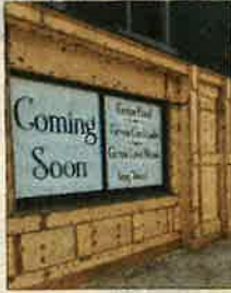
A work in progress: the exterior of the new Browne's - The Venue, which is expected to open in Tullamore later this summer
