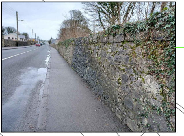
8A/B - BLOCKED/INSUFFICIENT DRAINAGE ALONG ROAD RESULTS IN LOCALISED SPLASHING OF PONDED SURFACE WATER ON THE ROAD AND FOOTPATH ONTO WALL FROM PASSING CARS. THIS CONTRIBUTES TO THE WIDER WEATHERING OF THE MASS CONCRETE WALL AND THE WASHING OUT OF MORTAR ALONG THE PROTECTED RANDOM RUBBLE STONE WALL. LONG TERM MAINTENANCE OF DRAINAGE ALONG ROAD REQUIRED.
