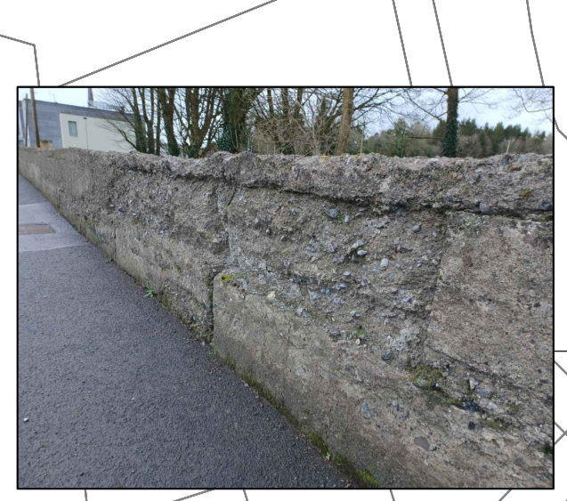
4B - FULL HEIGHT VERTICAL CRACK INDICATING LATERAL MOVEMENT OF WALL ALONG CONSTRUCTION JOINT
