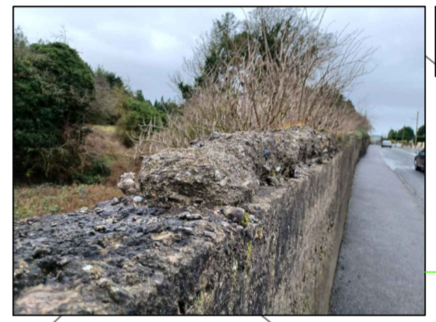
6 - MULTIPLE AREAS OF MISSING/ EXCESSIVELY WEATHERED/SPALLED COPING ALONG MASS CONCRETE WALL
