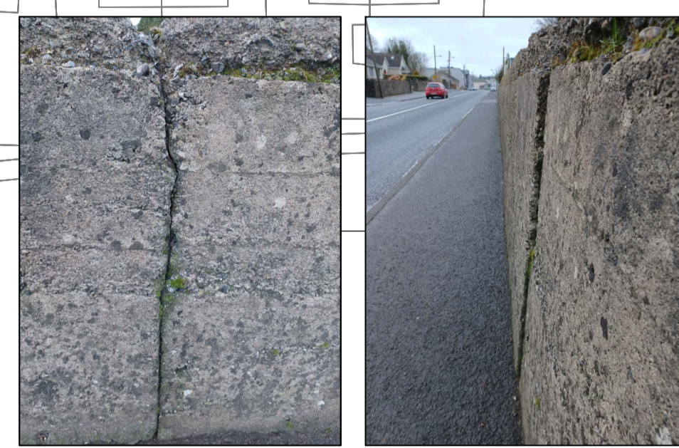
6 - MULTIPLE AREAS OF MISSING/ EXCESSIVELY WEATHERED/SPALLED COPING ALONG MASS CONCRETE WALL
