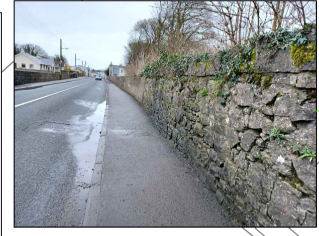
8A/B - BLOCKED/INSUFFICIENT DRAINAGE ALONG ROAD RESULTS IN LOCALISED SPLASHING OF PONDED SURFACE WATER ON THE ROAD AND FOOTPATH ONTO WALL FROM PASSING CARS. THIS CONTRIBUTES TO THE WIDER WEATHERING OF THE MASS CONCRETE WALL AND THE WASHING OUT OF MORTAR ALONG THE PROTECTED RANDOM RUBBLE STONE WALL. LONG TERM MAINTENANCE OF DRAINAGE ALONG ROAD REQUIRED.
