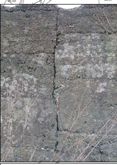
4A - HORIZONTAL AND VERTICAL CRACKS AT CONSTRUCTION JOINTS
