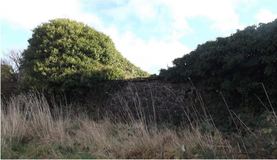
Fig. 7. Boundary wall on eastern boundary of site with mature Ivy shown.
