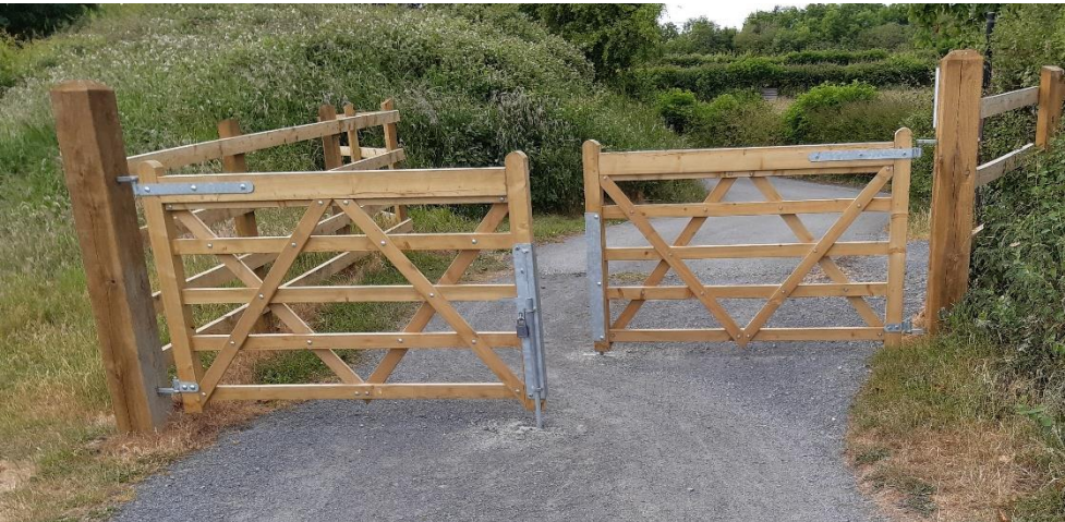
TYPICAL STAGGERED GATES
