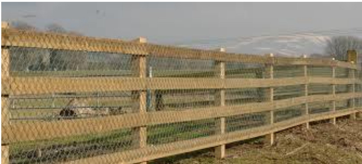
TYPICAL FENCING & GATES.
