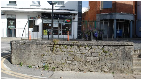
Rubble Wall and more modern railings LHS
