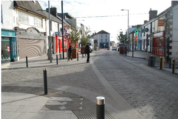
Approach looking east to Mardyke Street
