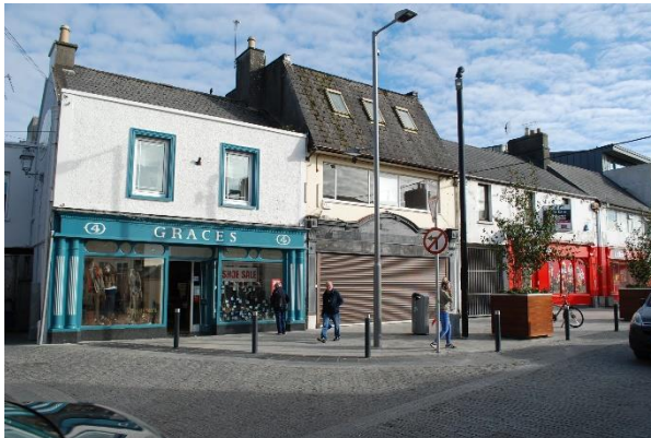
End of terrace to NW of Mardyke Street
