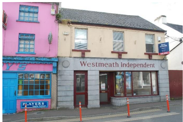
Two storey adjacent
