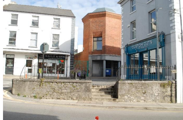
Raised area bounded by wall
