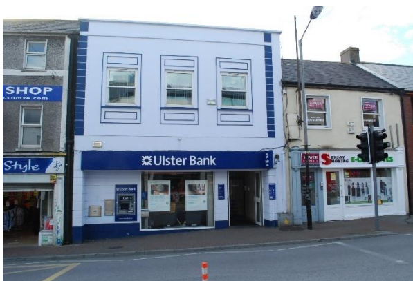
Tall 2 storey bank building
