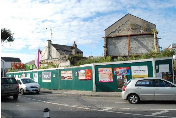
Hoarding to vacant site
