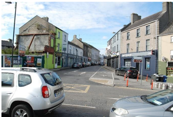
View looking west along Mardyke Street
