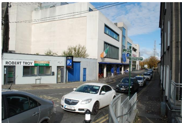
View looking North along Gleeson Street (LHS)
