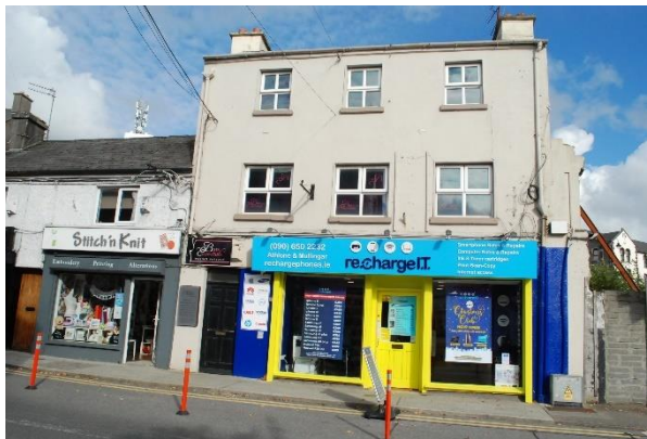
End terrace adjacent to vacant site (RHS)
