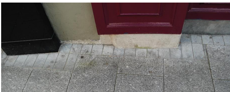
Important transition of larger format paving to smaller units at edges
