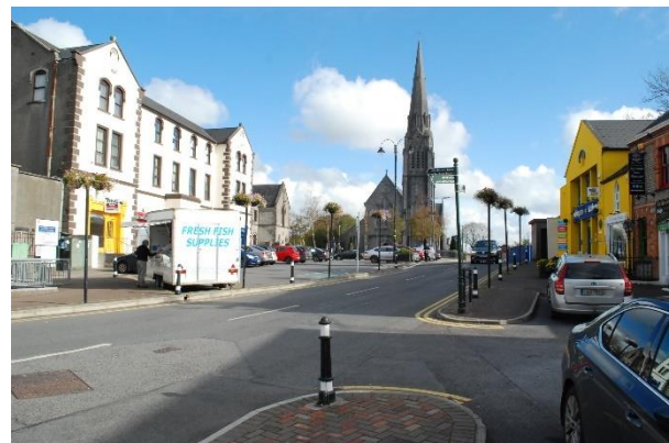
Surface parking to St Mary's Square
