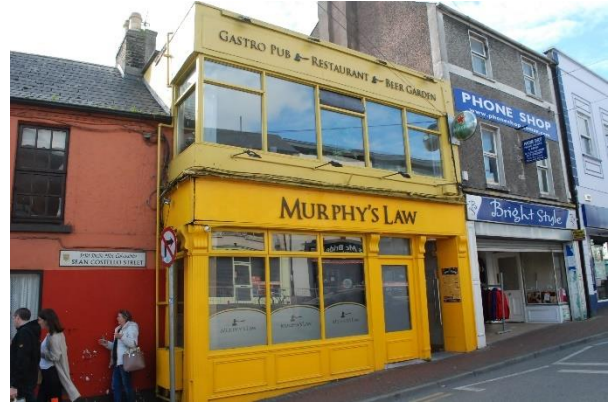
Much altered building
