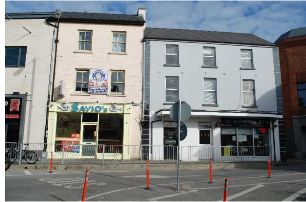
'Town Centre' scaled with building to the RHS
