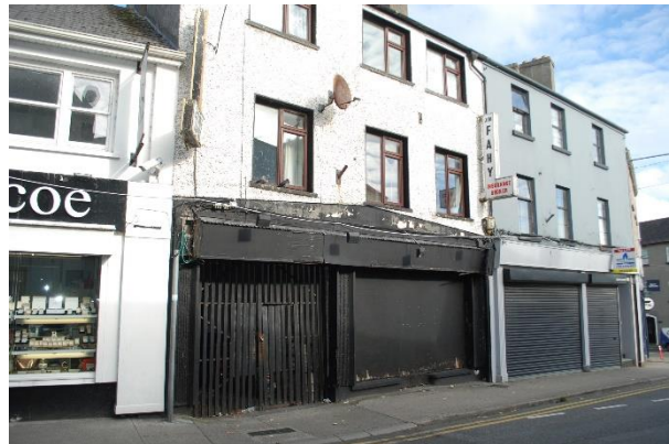
3 storey building adjacent - altered
