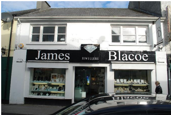
Typical traditional 2 storey building altered
