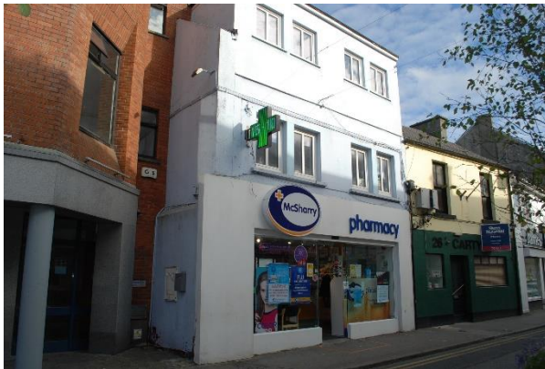
Raised 3 (previously 2) storey building
