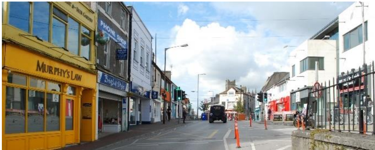
Widening of street at junction with Mardyke Street
