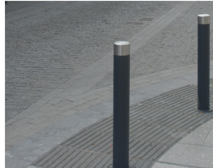
Change in materials and use of bollards to delineate road edges.
