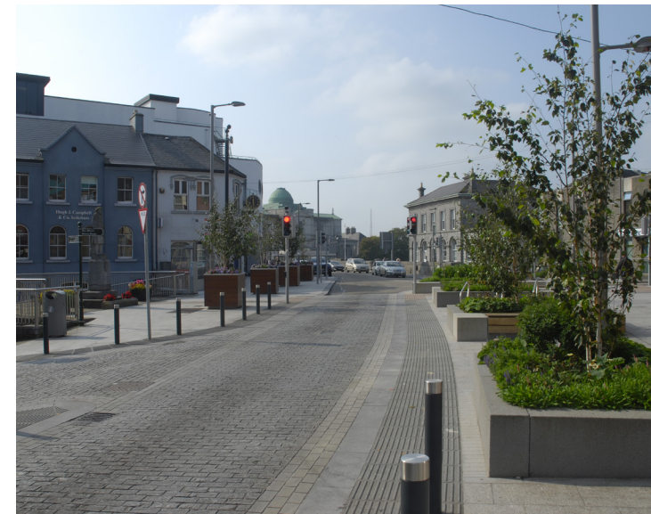
Public space with street furniture; raised planters, seating edges and bike stands.
