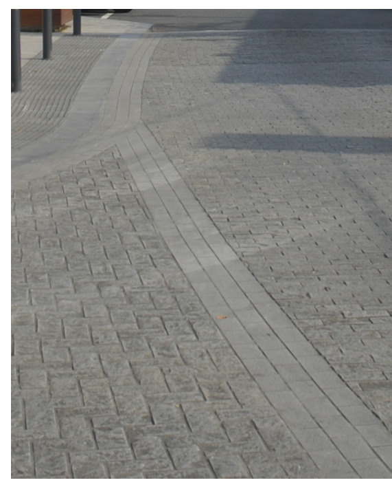
Granite paving and feature band on Church Street
