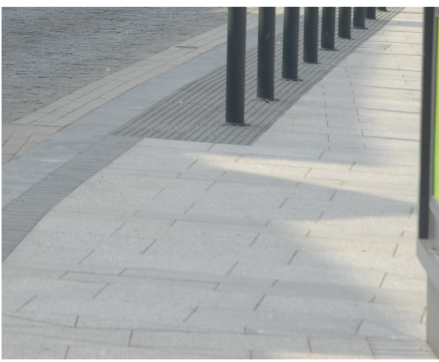
Granite paving and tactiles on Church Street
