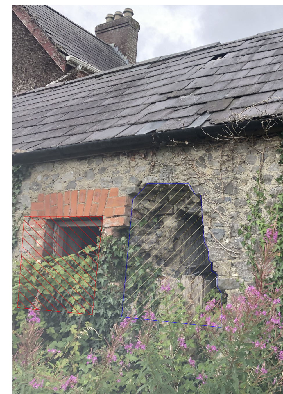
WIDENING EXISTING OPENING / EXISTING OPENING TO BE REPAIRED WITH SALVAGE STONE
