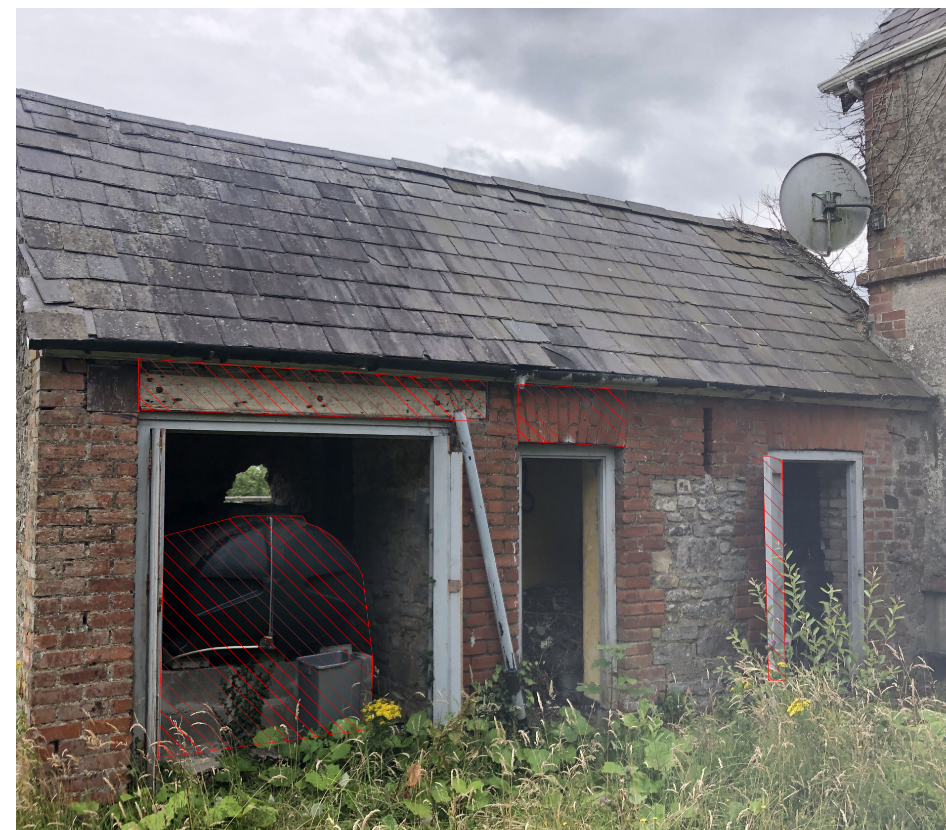
OIL TANK TO BE REMOVED / EXTERNAL DOORS TO BE REPLACED / INCREASING EXISTING OPENINGS
