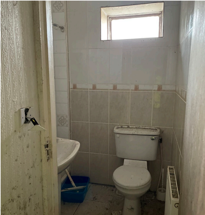
Fig 67: Internal Elevation 9.A. Existing toilet.
