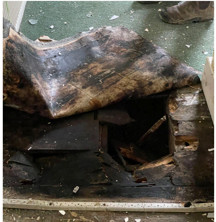
Fig 35: Internal Elevation: Timber floor with carpet. Threshold from room 2 to room 3.
