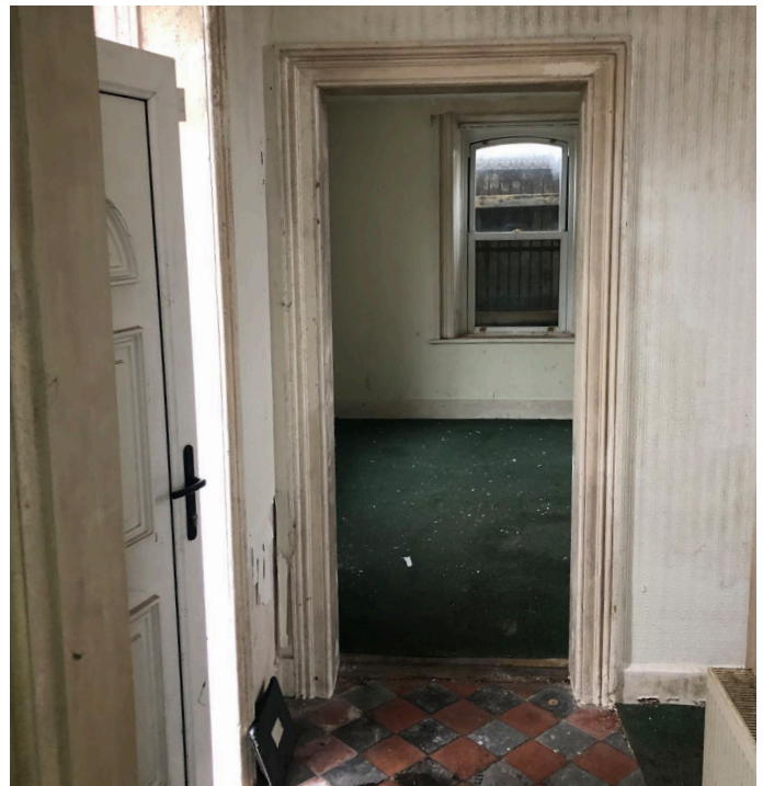
Fig 23: Internal Elevation 1.D. Doorway to Room 2.
