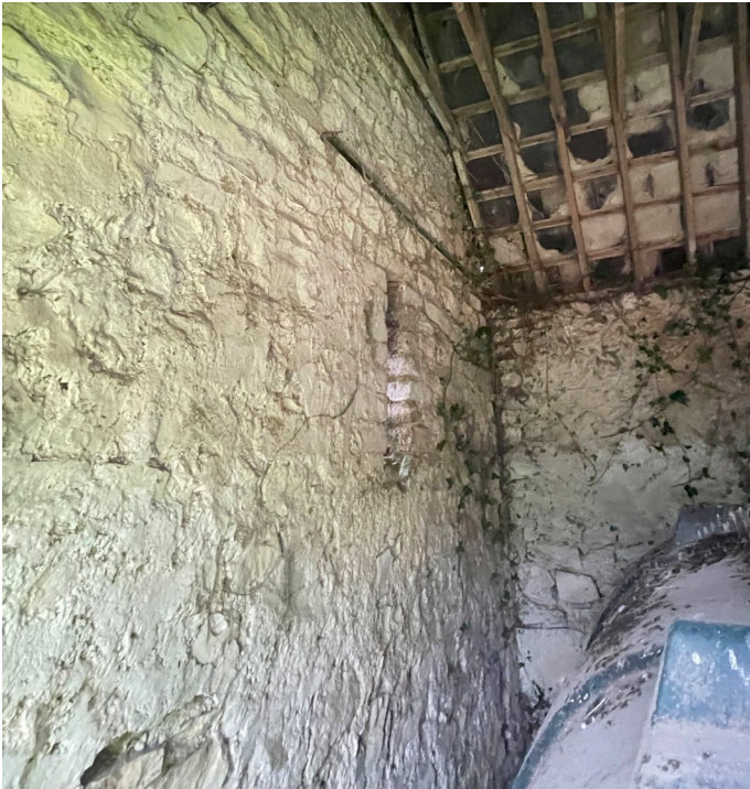
Fig 57: Internal Elevation 6.A. Stone Wall.
