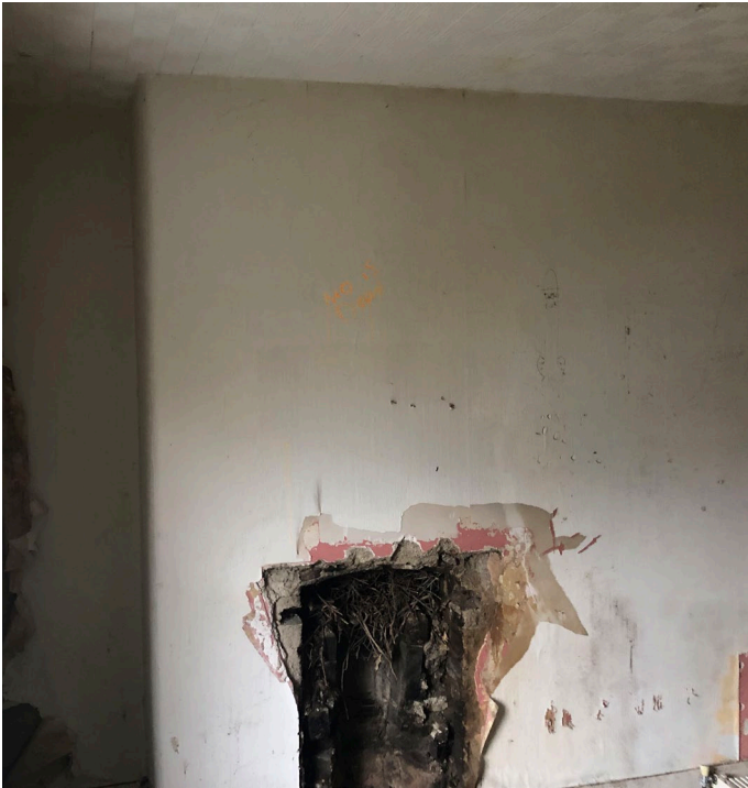
Fig 73: Internal Elevation 11.A. Fireplace opening.
