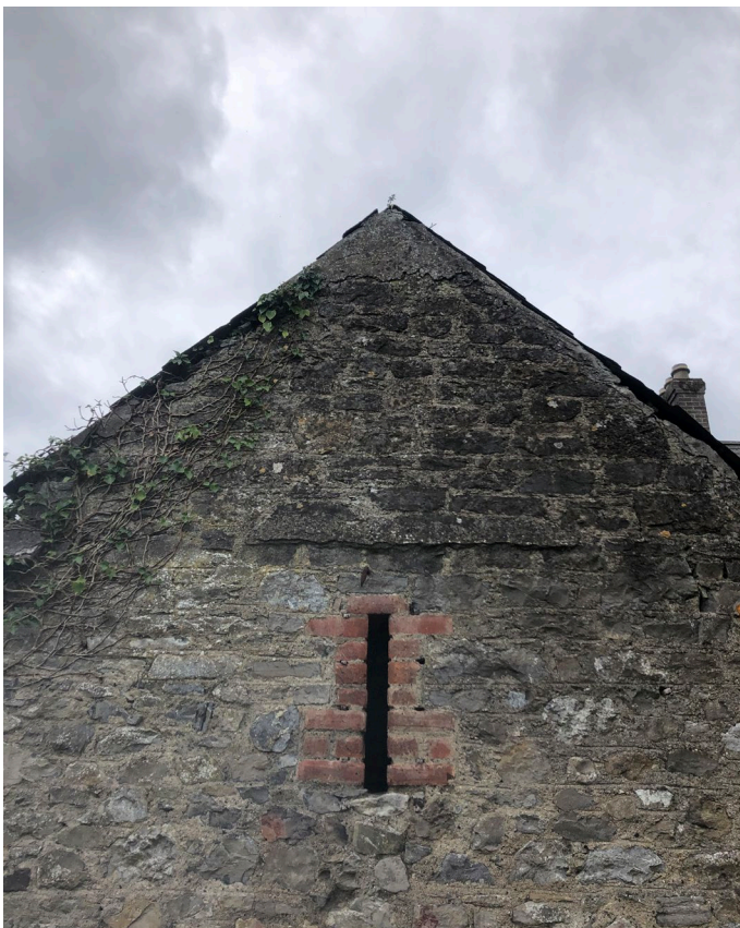
Fig 10: Elevation B extension. Opening to stone wall. *Note picture was taken in March 2024.
