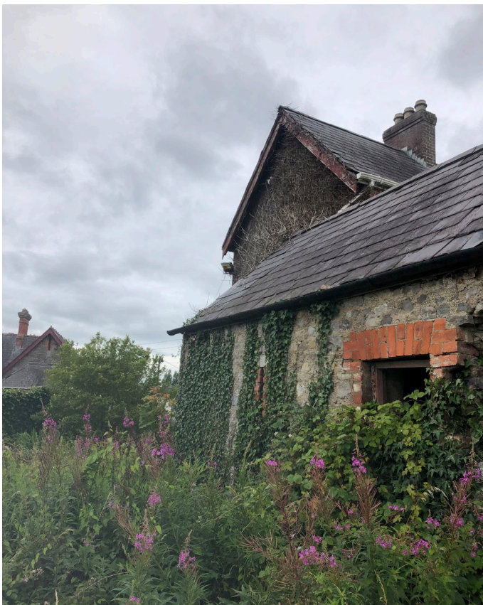
Fig 18: Elevation D. *Note picture was taken in July 2020.
