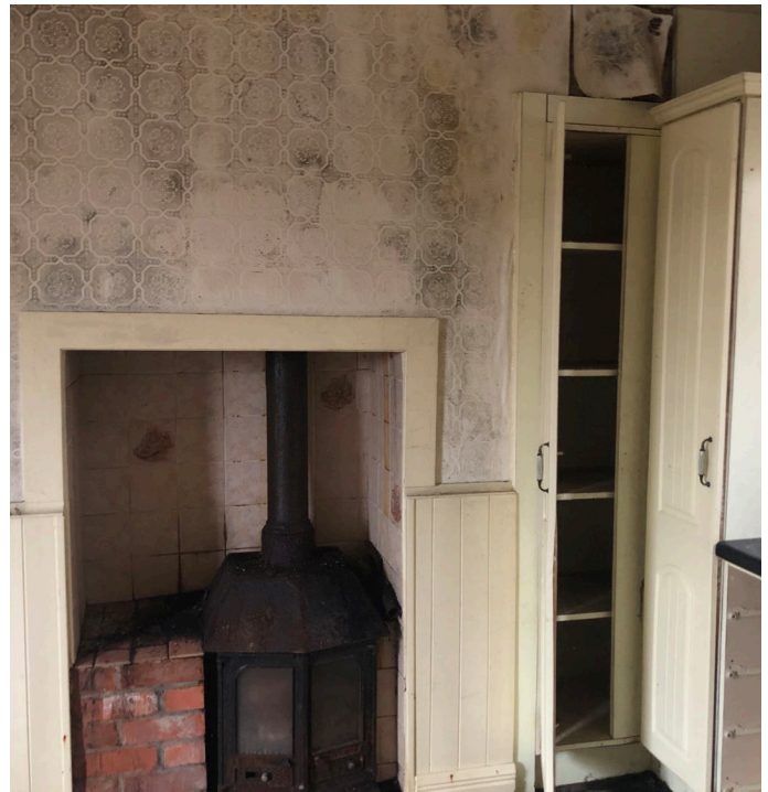
Fig 41: Internal Elevation 3.C. Existing iron stove and cabinets.
