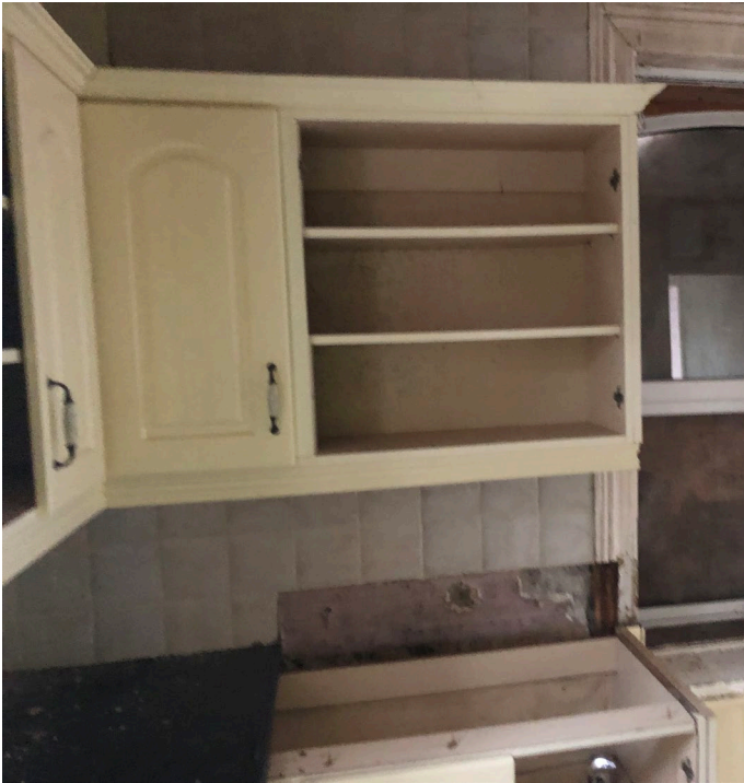
Fig 36: Internal Elevation 3.A. Kitchen cabinets.
