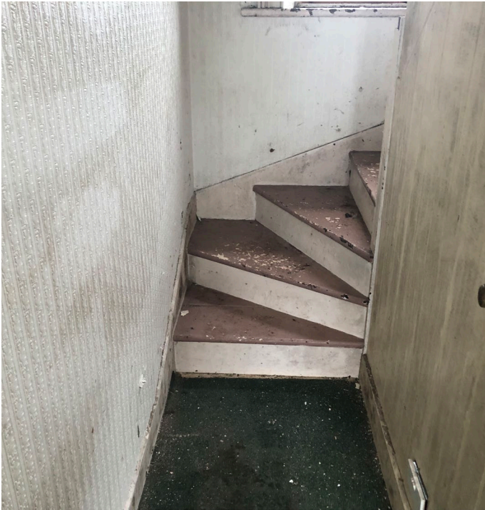
Fig 24: Internal Elevation 1.A. Staircase.
