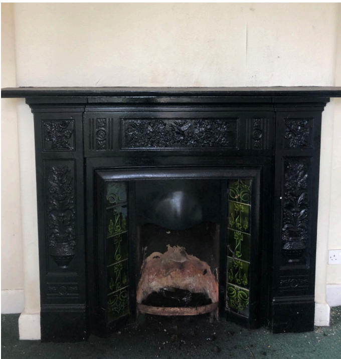
Fig 53: Internal Elevation 4.D. Detail of existing fireplace.
