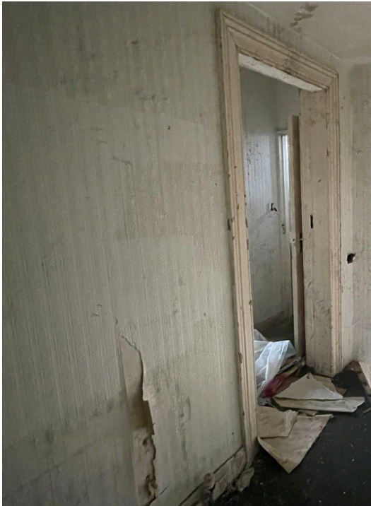
Fig 65: Internal Elevation 7.D. Doorway to room 8.
