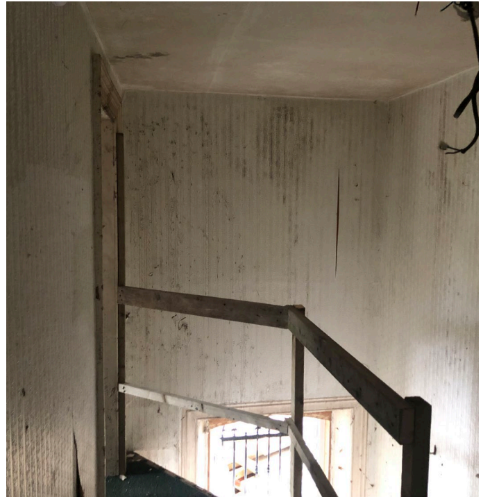
Fig 66: Internal Elevation 7.D. Temporary timber railing.
