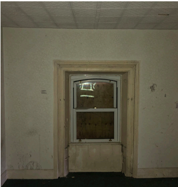
Fig 79: Internal Elevation 12.C. Existing window boarded up.
