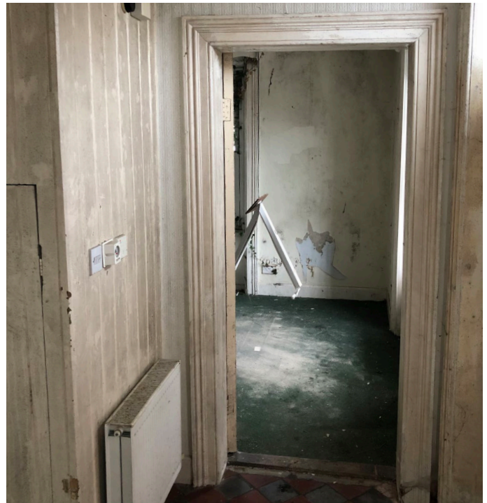
Fig 21: Internal Elevation 1.B. Doorway to Room 4.
