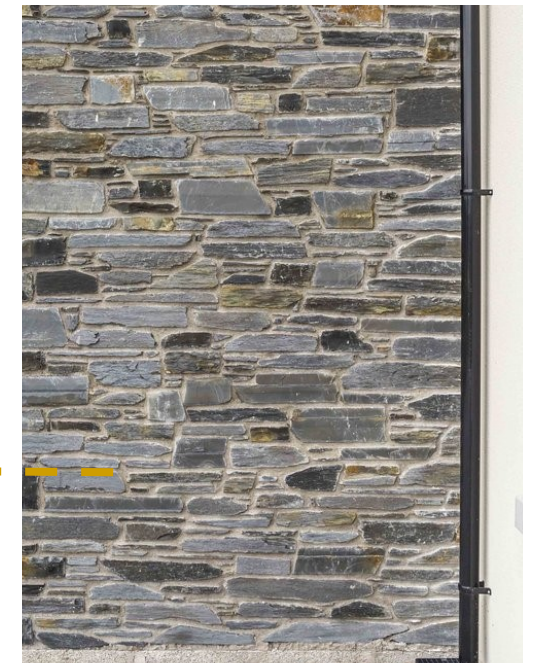
Local Limestone external cladding to Shop front & gable end.
