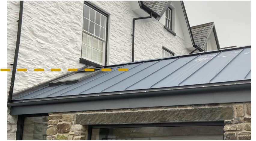
Zinc Standing Seam roofing and close fascia to new rear extension
