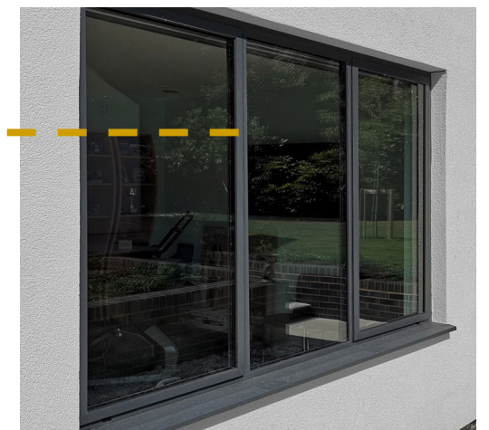
Aluminium Windows & Doors to new extension / Rear
