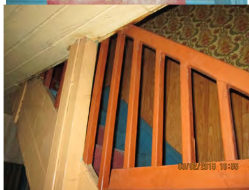
Interior — Stairs detail.
