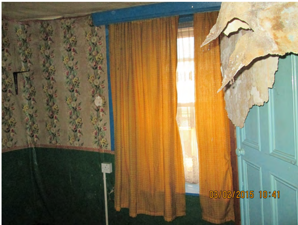
Interior — First Floor Bed 1 to front elevation
