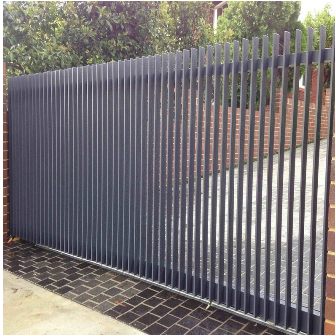
Slatted Steel gate and fence wall as security to rear of property.
