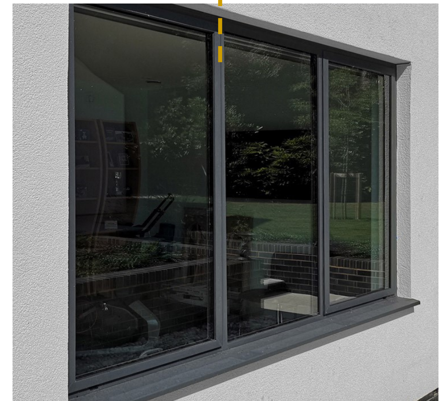
Aluminium Windows & Doors to new extension / Rear
