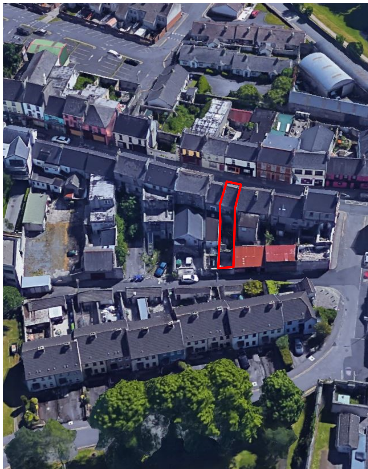
Aerial Photo—Site Location—From South to North
