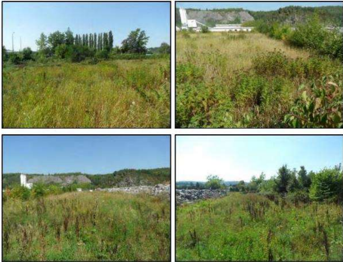
Figure 84: Photos of developments at the power plant site and on the Natagora plot (Source: Electrabel S.A. 2017)
