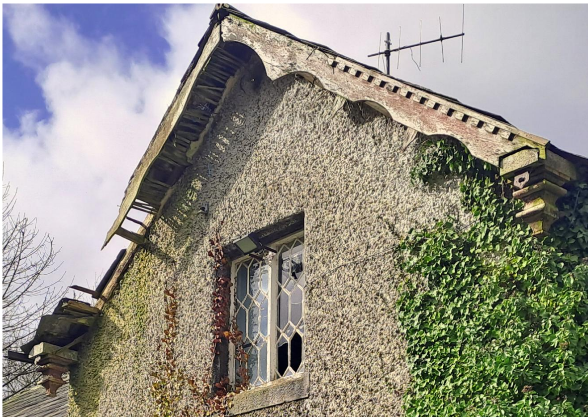
A08: Roof Barge Boards and Lanterns
