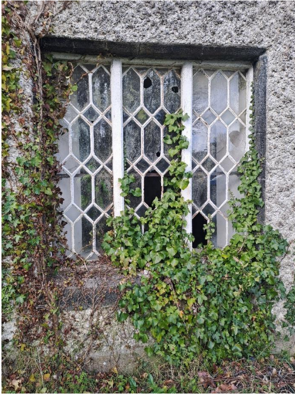
A06: Window Tracery & Limestone Features
