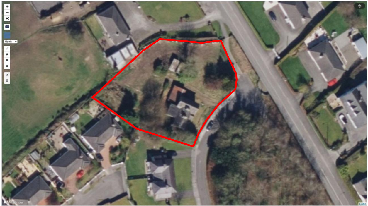
Figure 3 Image of Site
