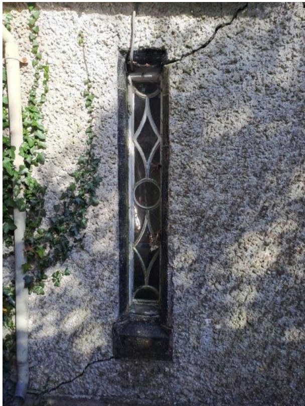
A14: Lancet Window with Metal Tracery
