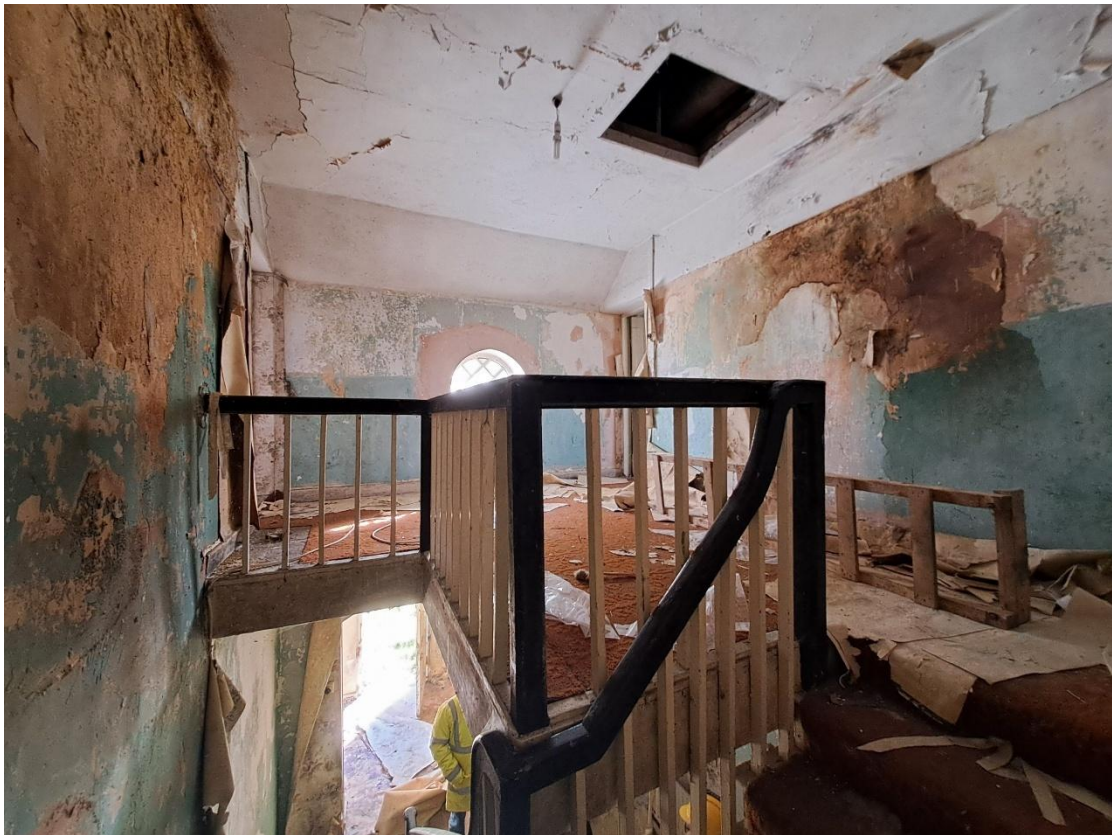
A11: Stair Landing and Railing
