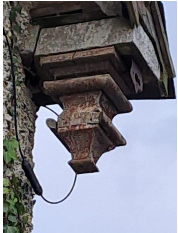
A15: Roof Barge Timber Lanterns
