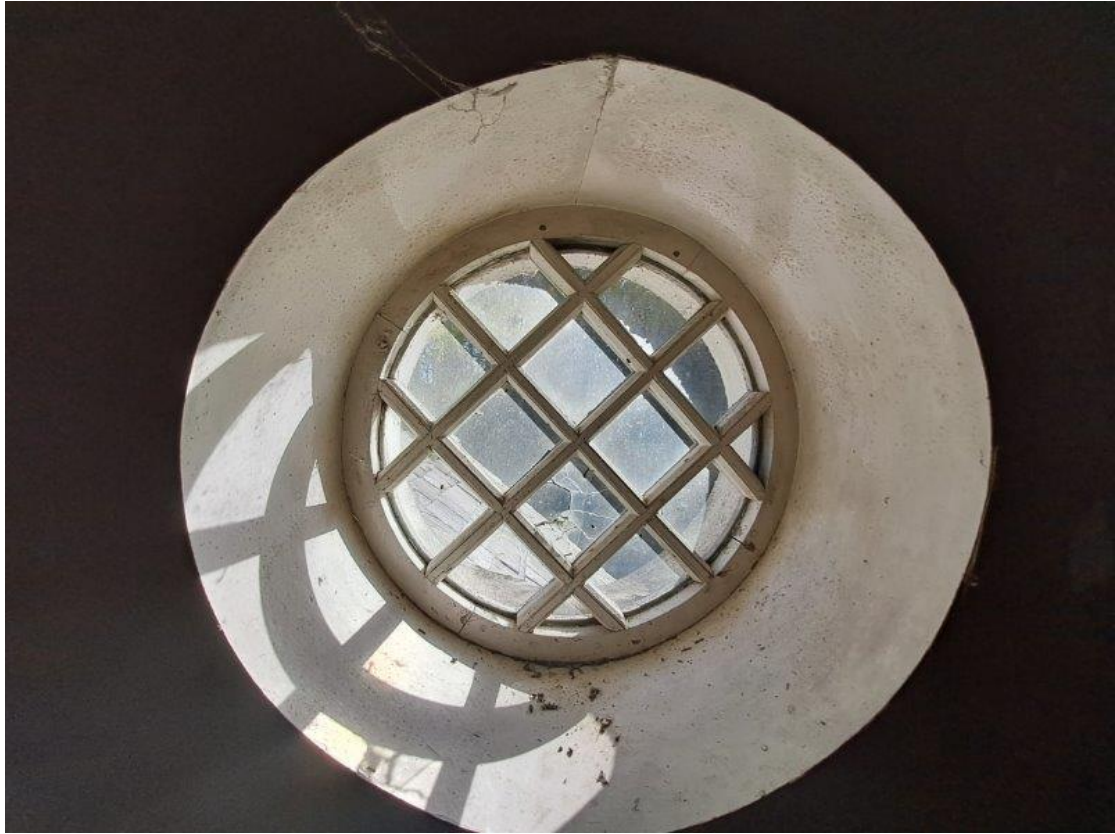
A16: Oculus window with timber tracery
