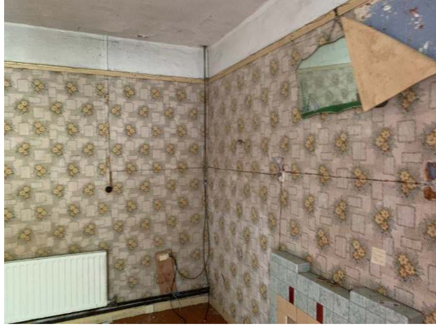
Photo 5 – Ground Floor Walls
