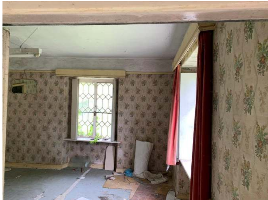
Photo 6 – Ground Floor Walls
