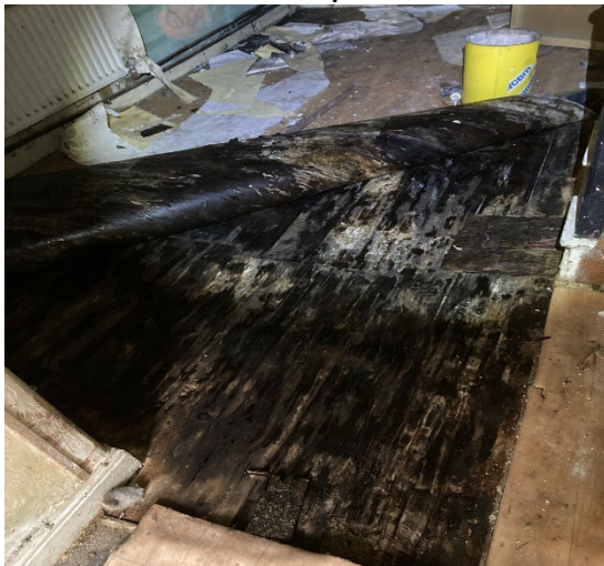
Lino on top of rotten timber in the ground floor hallway. Lino over concrete floor tiles inside the front door.
