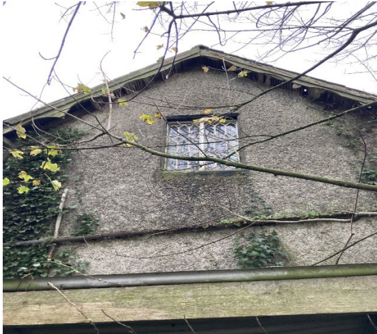
Side elevation over the car port. The fascia was timber.
