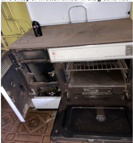
Kitchen cooker. No rope seal present.
