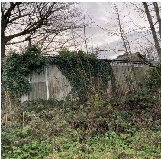
Detached outhouse inside and outside.
