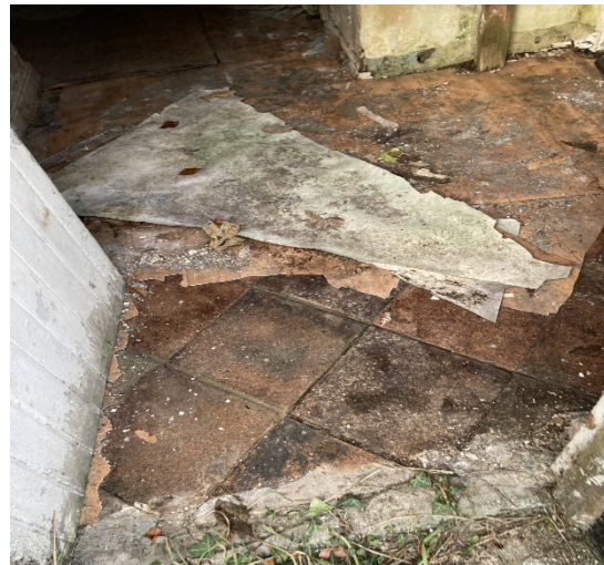
Lino on top of rotten timber in the ground floor hallway. Lino over concrete floor tiles inside the front door.
