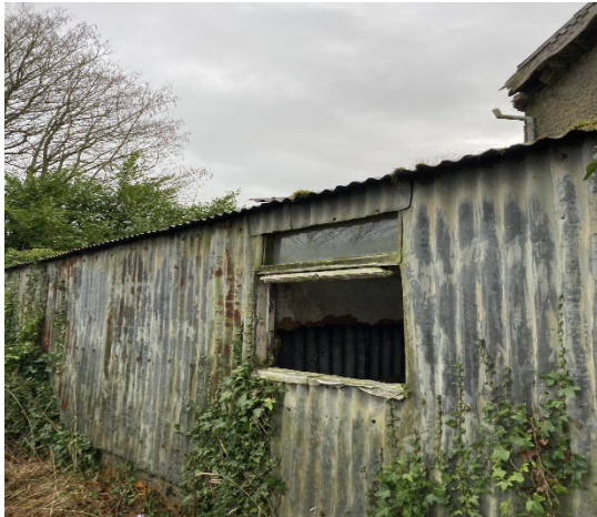
Lean too outhouse inside and outside.
