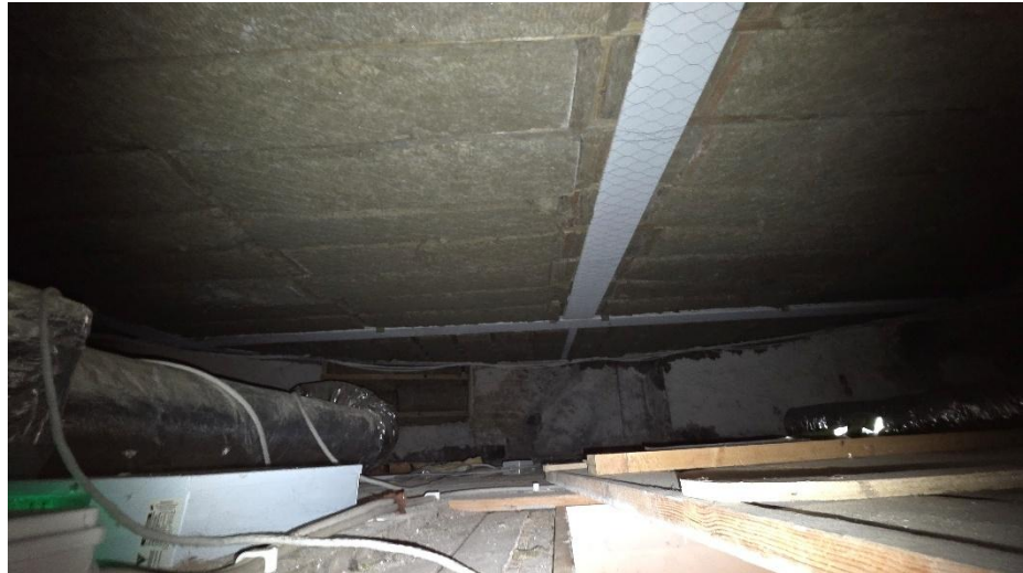
Figure 13: View inside void of underside of 2012 floor structure
