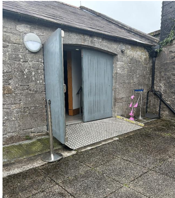
Figure 19: Access to Terrace from Armoury
