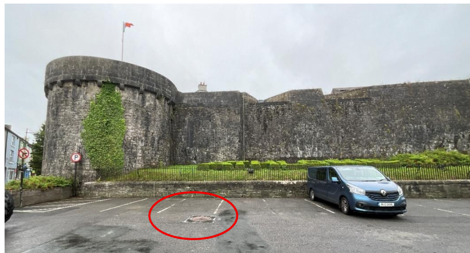
Figure 6: Public Sewer manhole circled
