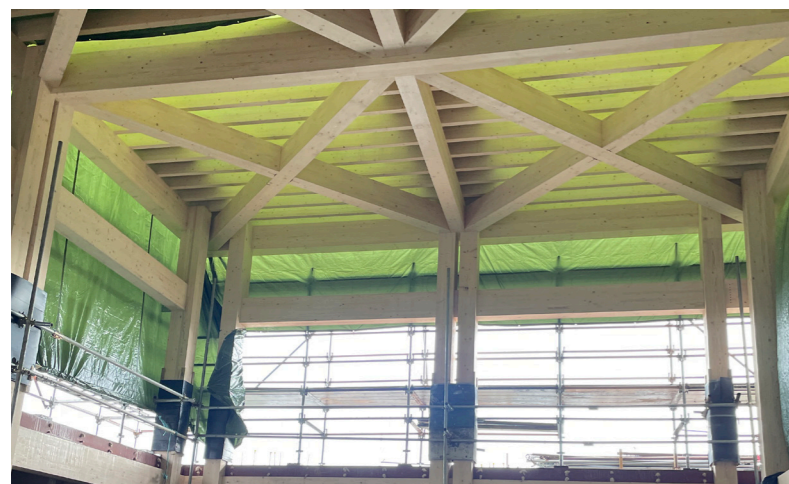
Fig. 14 Construction of proposed library on site 16.02.24
