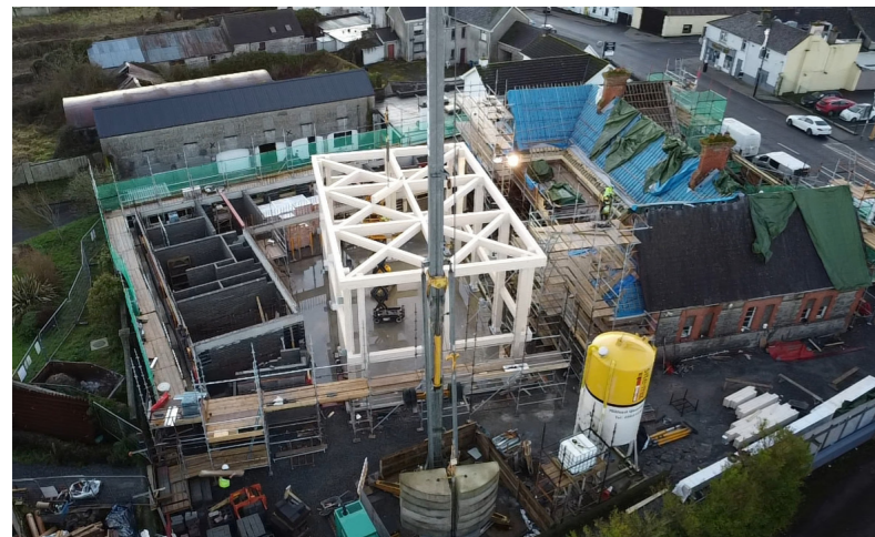
Fig. 13 Construction of proposed library on site 13.12.23
