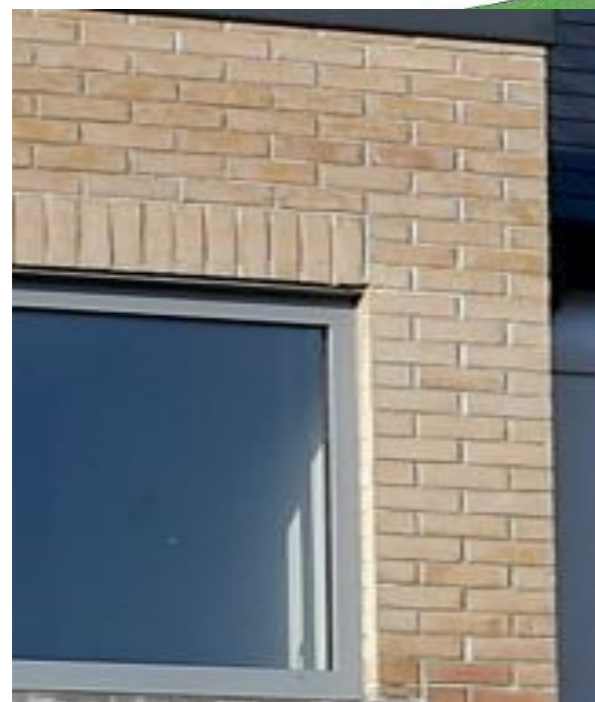
Selected quality buff coloured Brick by King-court or similar supplier with textured finish
