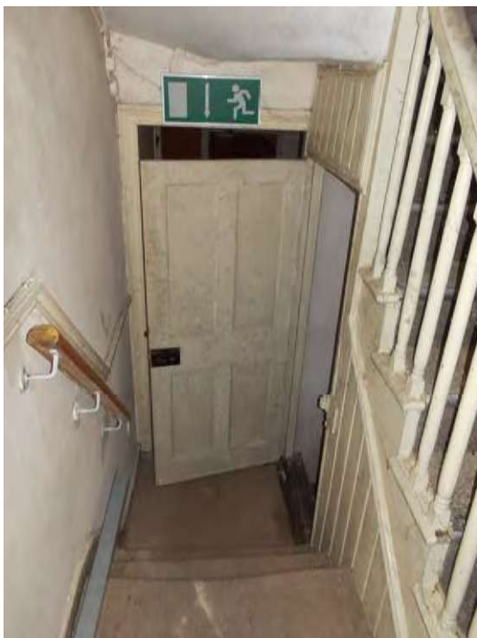
Interior—Ground Floor Stairs / Lobby
