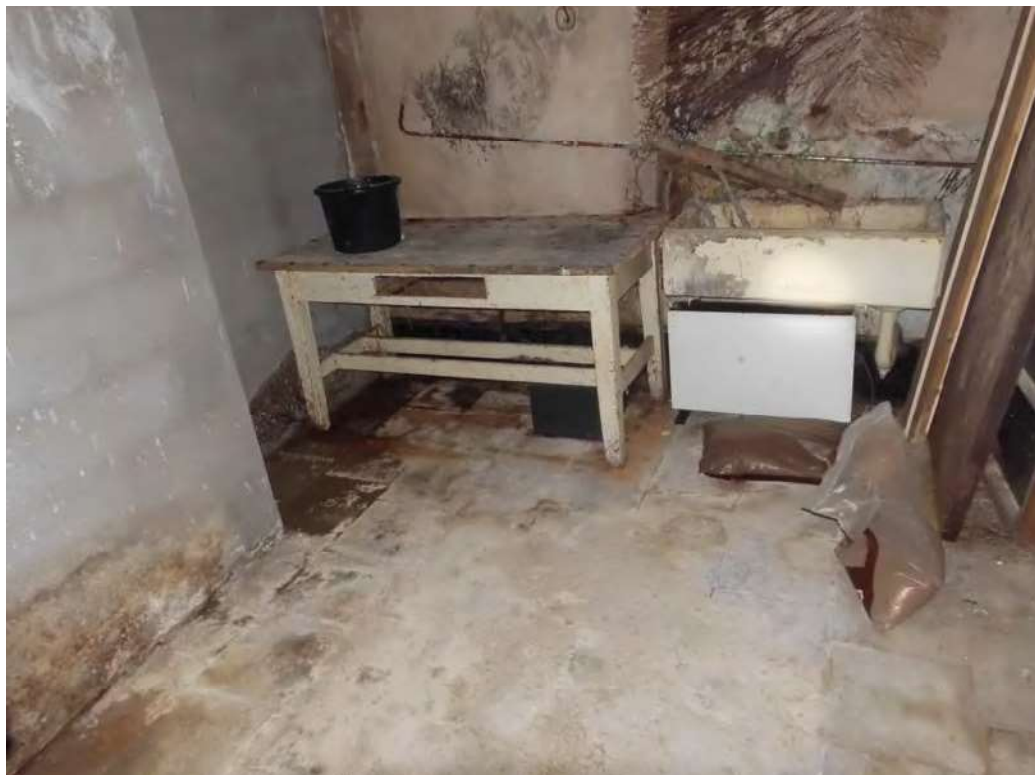
Basement —View rear Room.
