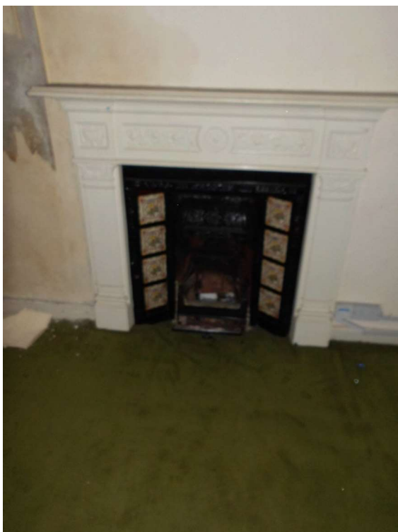
Interior— Detail Cast Iron Fire Surround
