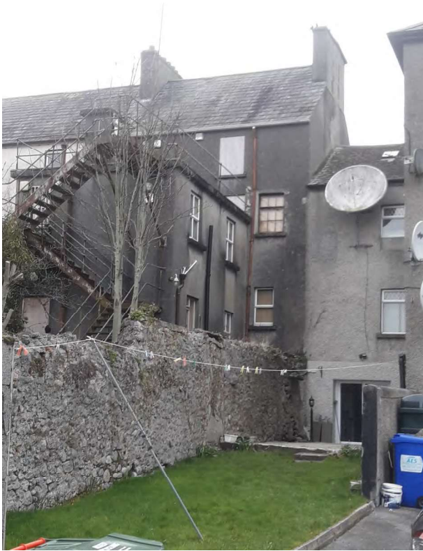
Exterior —Rear Elevation S
