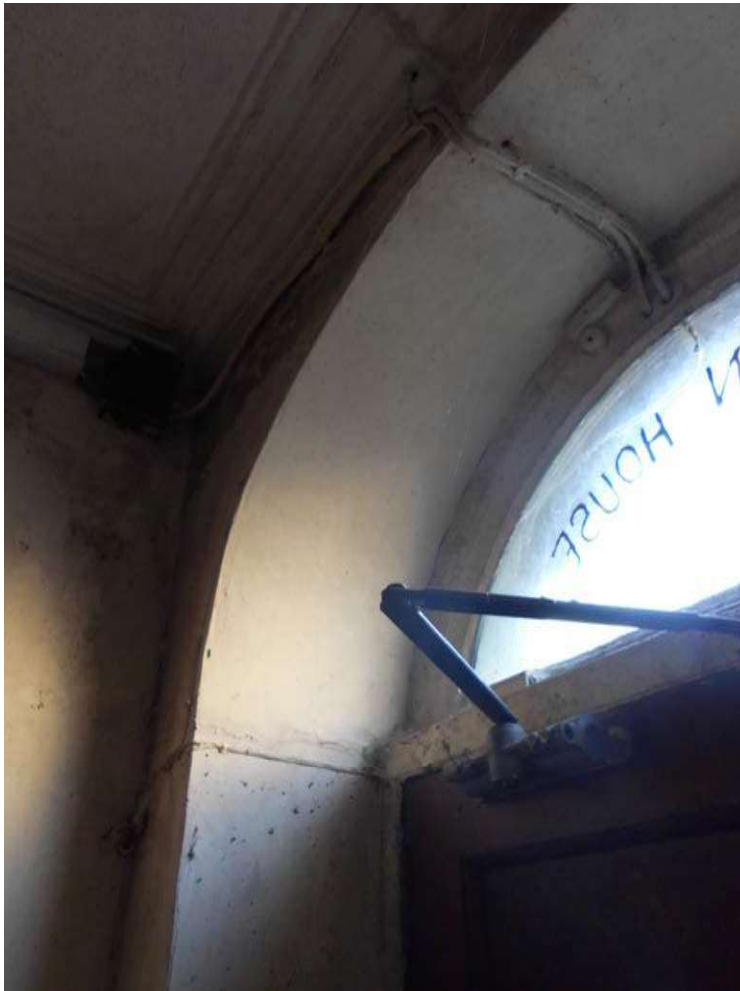
Interior—Ground Floor Front Entrance Detail
