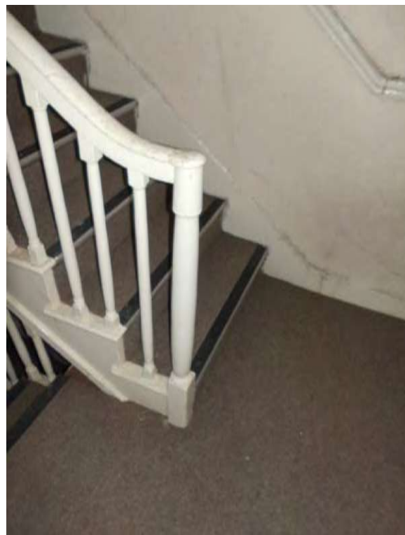
Interior— Detail Stairs.
