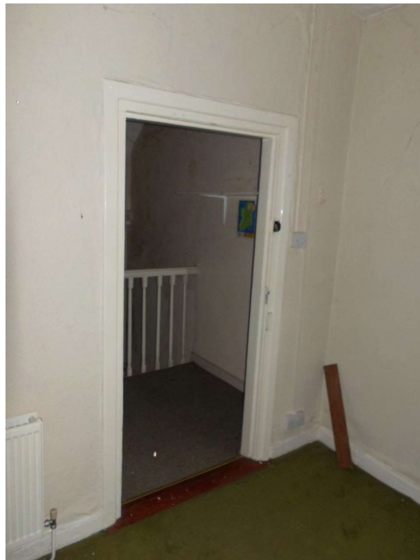
Interior—Second floor Front Room view to Landing
