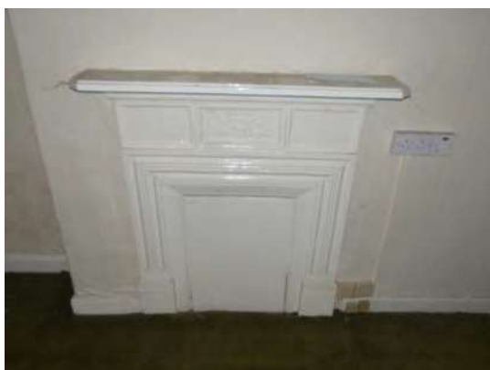
Interior detail —Second floor Front Room view to cast iron fire surround.
