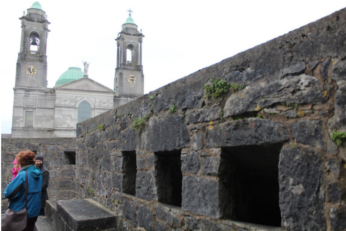
The entrance ramp and pistol loops date from the Napoleonic stage of development 1800-1827.
