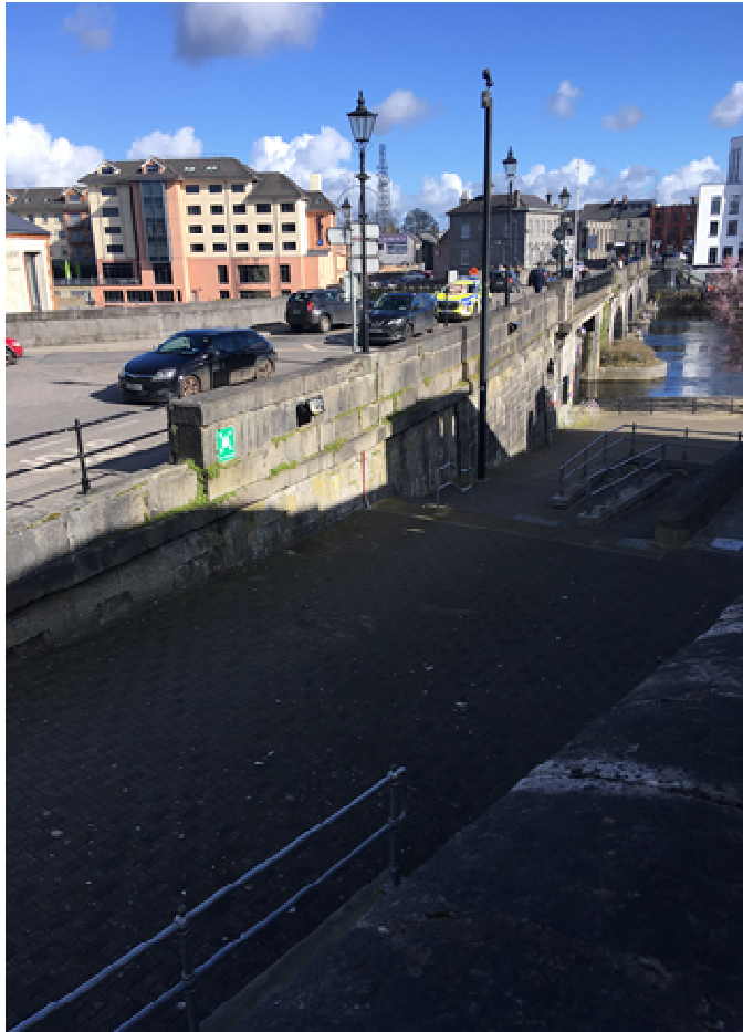
Plate 1: Pedestrianised space to the north of castle, facing east
