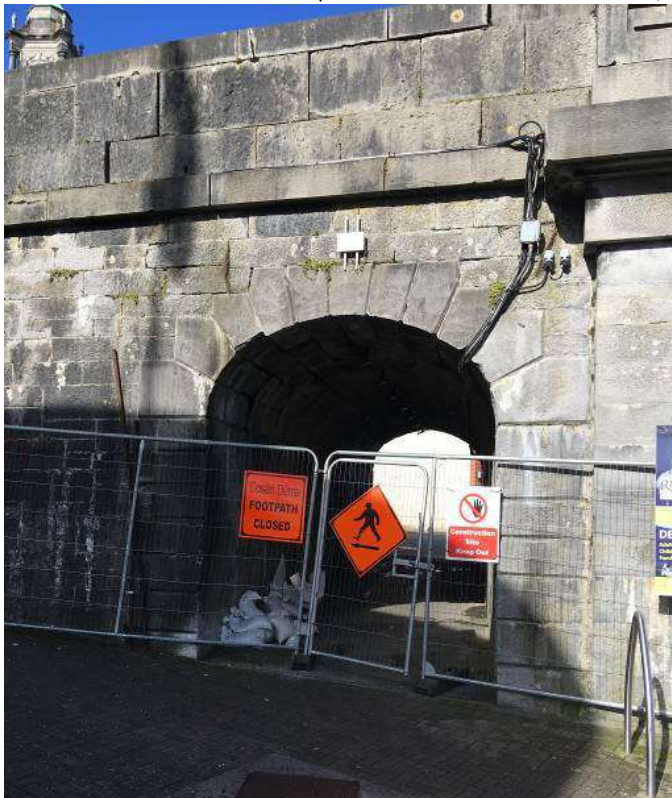
Plate 2: Pedestrian underpass, facing north-northwest
